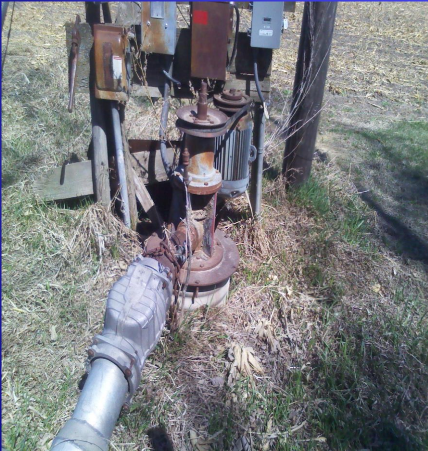
Belt Drive Gear Head
