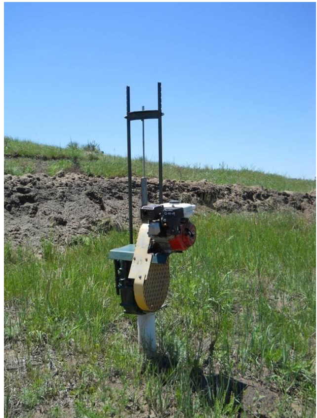
Groundwater monitoring well at Crow Butte Resources Inc., Dawes County.
