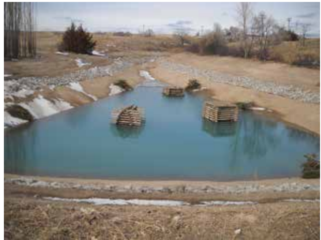
Newly installed habitat structures to enhance the fishery, Big Springs Community Lake, Deuel County..
