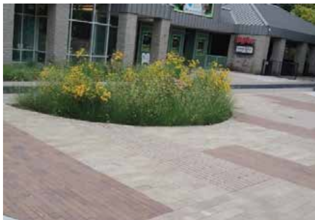
Permeable pavers installed at Lincoln Children's Zoo.
