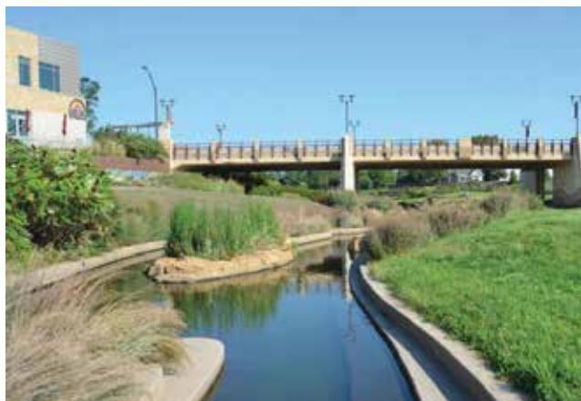
Antelope Creek open channel near Union Plaza.
