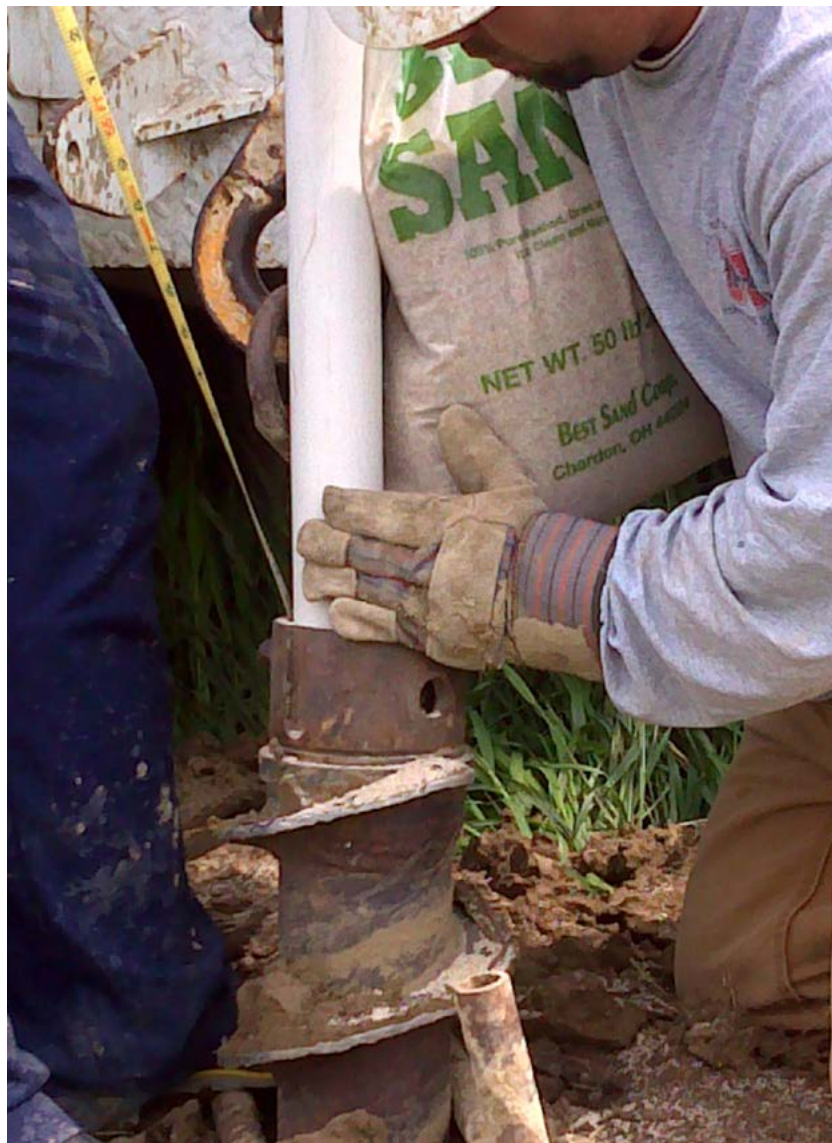
Installing a monitoring well near Clearwater, NE.
