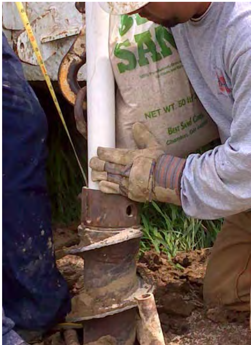
Installing a monitoring well near Clearwater, NE.
