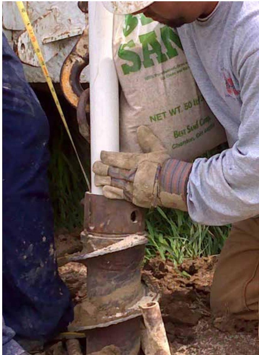
Installing a monitoring well near Clearwater, NE.
