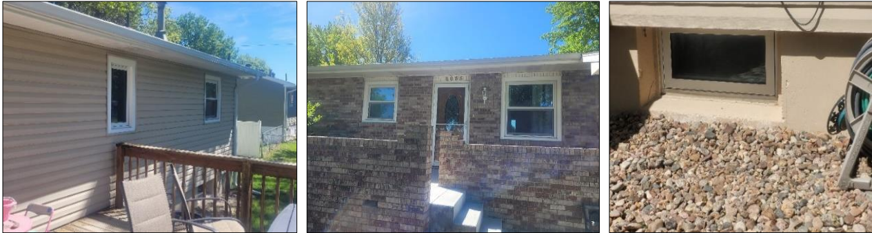
New energy efficient windows installed with funds from the NDEE's Dollar and Energy Saving Loan Program (2023).
