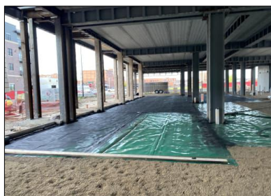
Vapor mitigation system granular layer and membrane
