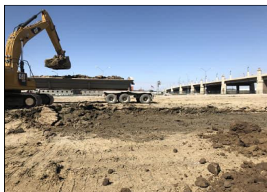
Excavation and disposal of contaminated soil
