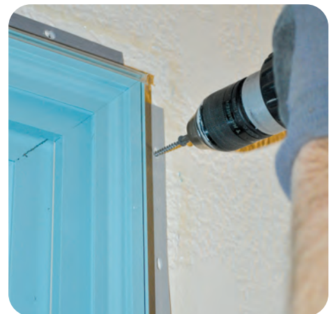
6. Level the window using shims and secure with mechanical fasteners
