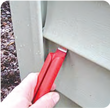
4. Remove siding as needed
