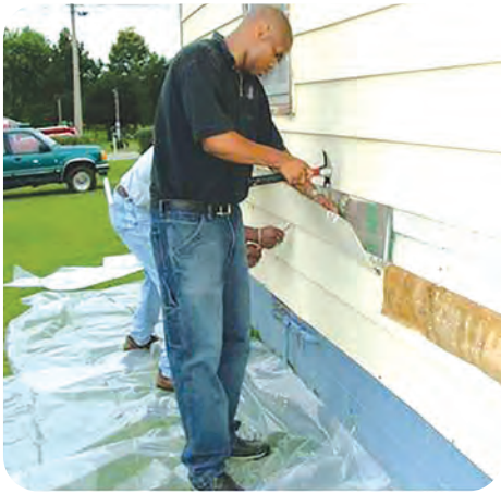
1. Protect work area from debris and dirt
