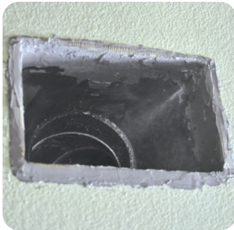
D-4. Apply mastic over mesh and allow to dry completely before reinstalling register
