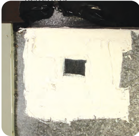
C-2. Cut patch that will extend over entire gap or hole and affix with mechanical fasteners
