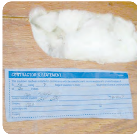
5. Fill cavity and leave appropriate documentation
