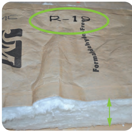
2. Insulation R-value matches work order
