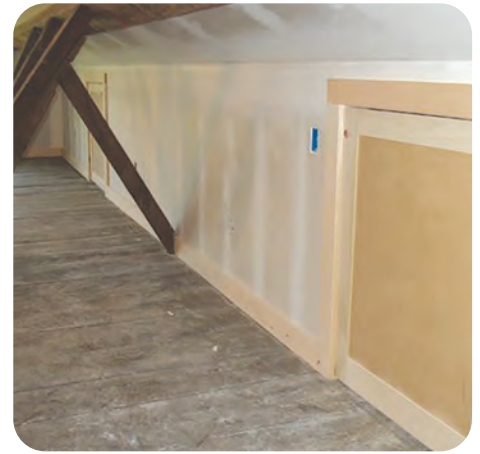
If space is used for utility access, storage, or permanently habitable, separate foam from the subspace with a suitable thermal barrier covering, such as 1/2-inch gypsum board
