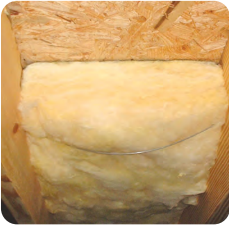
5. Batts are in good contact with subfloor
