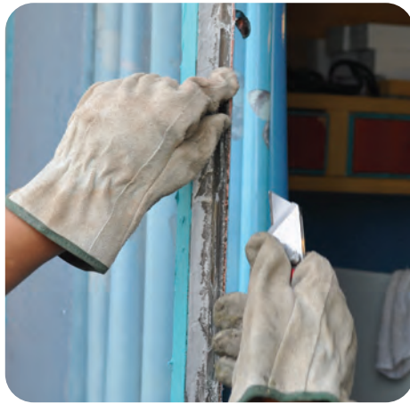
2. Clean all debris, caulk, etc., from sash
