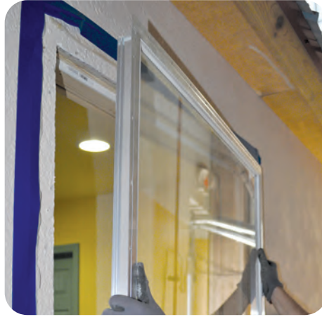
2. Remove existing window
