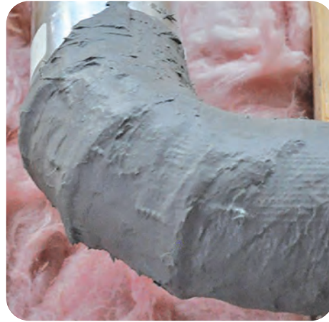
A-2. Apply mastic over all mesh tape and all gaps, seams, joints, etc.
