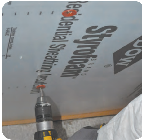
2. Attach rigid barrier to cover entire cavity
