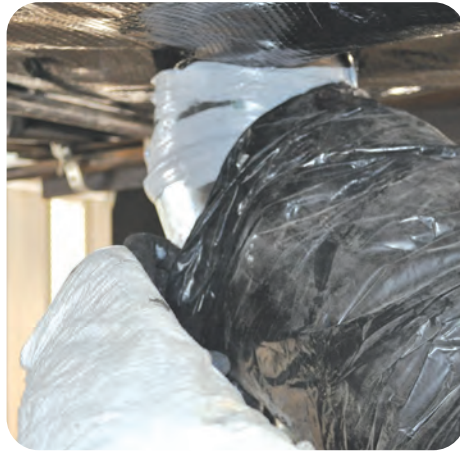
2. Pull insulation over hard connections as needed
