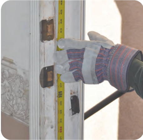
4. With threshold adjusted, measure door opening height
