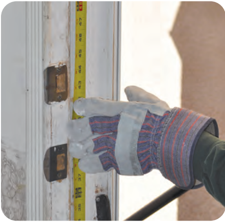
1. Measure doorway for weatherstripping
