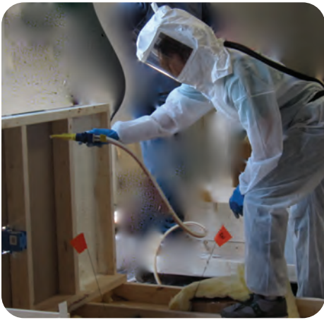
Ensure proper PPE when installing 2-Part Spray Foam
