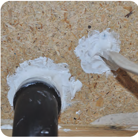
1. Verify all air sealing and prep work is complete
