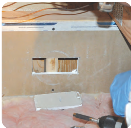
2. Cut holes in backing material to allow access to all cavities
