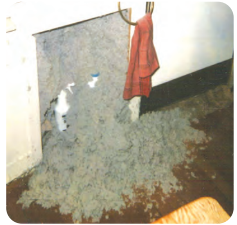
3. Ensure wall integrity is complete (no holes)
