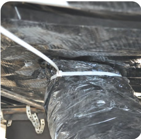
3. Secure vapor retarder layer at boots
