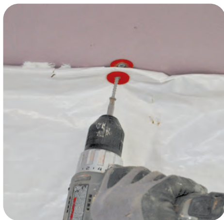
2. Attach new belly wrap
