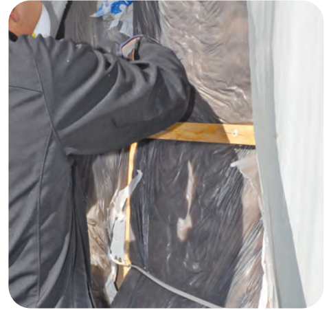
7. Gently tug batt into place and tuck remaining batt under lower belt rail and fit down to bottom of cavity with minimal compression
