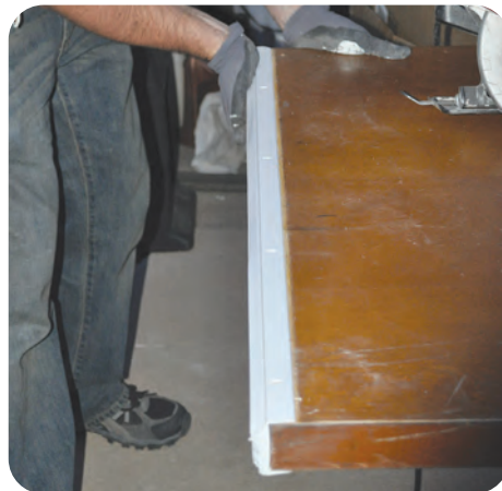
8. Ensure that door bottom sits tight against the door and reinstall door
