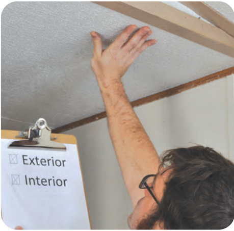
1. Verify integrity of ceiling to hold weight of insulation
