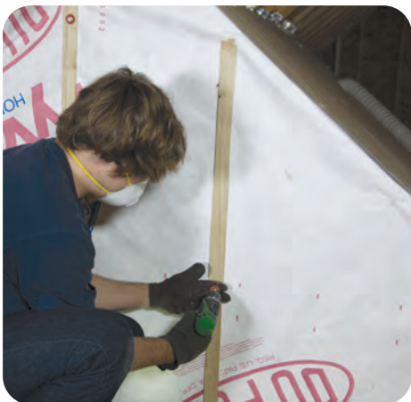
1. Securely install backing material over entire knee wall
