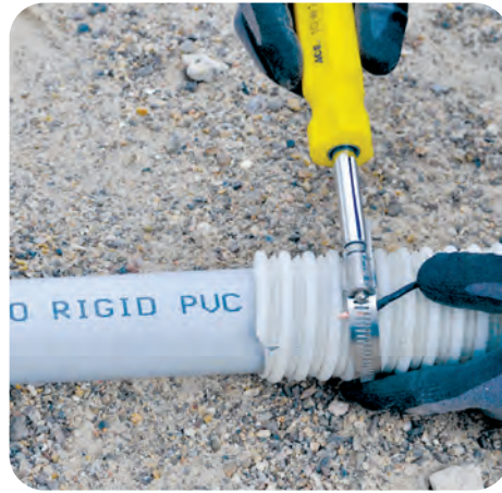
2. Ground blower hose to reduce chance of electrical build-up
