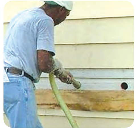
6. Fill cavities completely and to proper density
