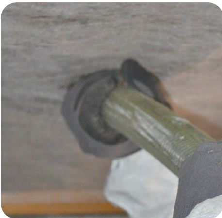
13. Loose fill netting to required density
