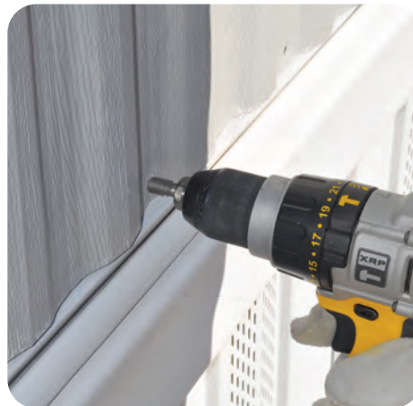
9. Reattach mechanical fasteners
