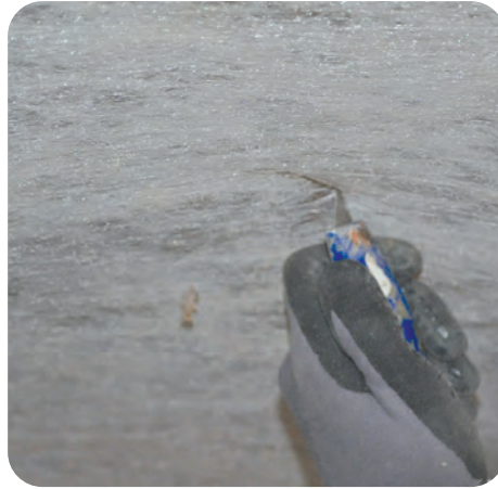
12. Cut access hole for fill tube
