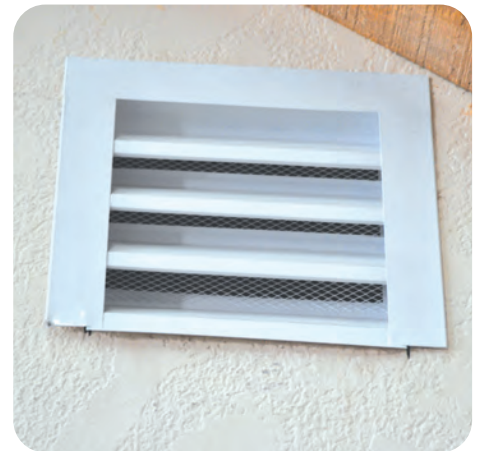
6. Reseal gable end or install gable vent at peak that has no more than 1/2 inch mesh screen. Repeat all steps from other end, if needed.
