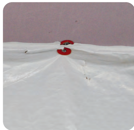
3. Seal seams of belly wrap
