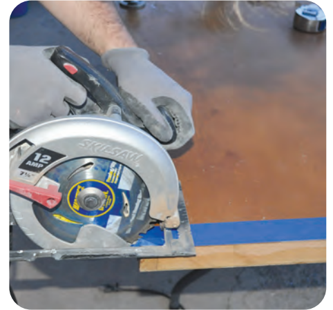
6. Trim door, if possible, to ensure good fit of door bottom
