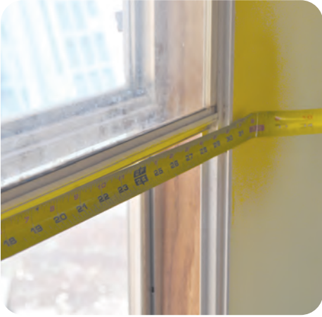
1. Measure window to be replaced
