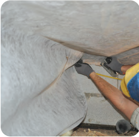
11. Cover the entire cavity to ensure continuous insulation coverage and prevent insulation from blowing out the ends
