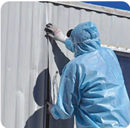
8. Reinstall siding
