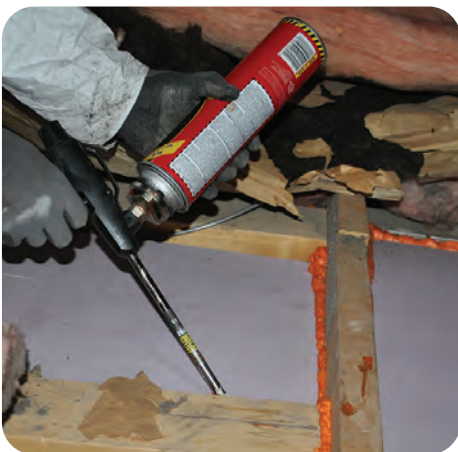
3. Ensure air sealing, if any, is completed
