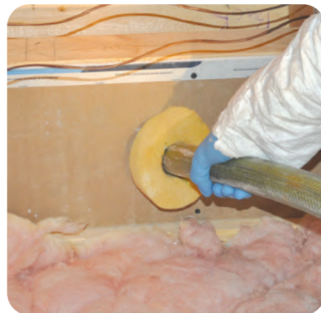
3. Blow insulation into cavities to meet dense-pack standards
