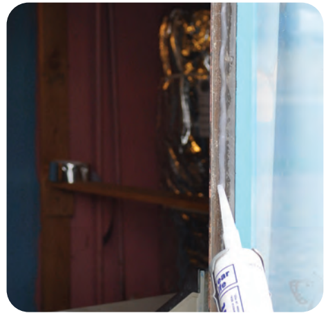
4. Run interior bead of caulk
