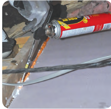
B-2. Seal around infill materials
