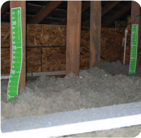
5. Depth rulers installed, 1 per 300 square feet
