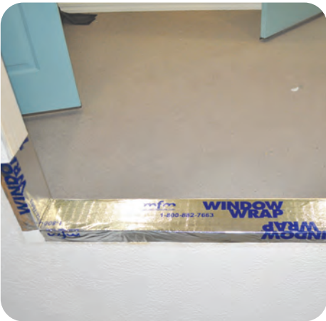
4. Replace flashing as needed
