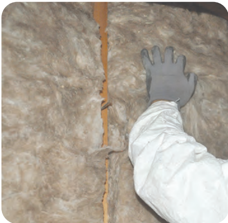
3. Install batts with minimal compression
