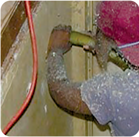
7. Dense pack stairway walls
