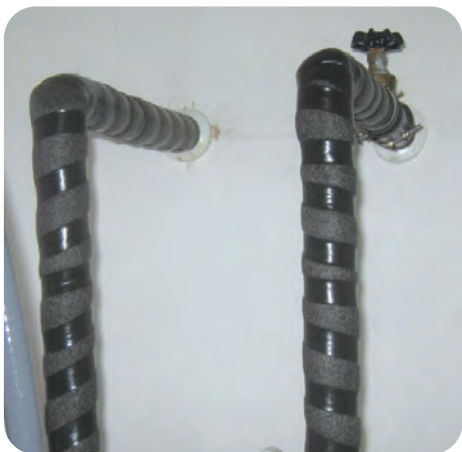
Secure seams with tape
