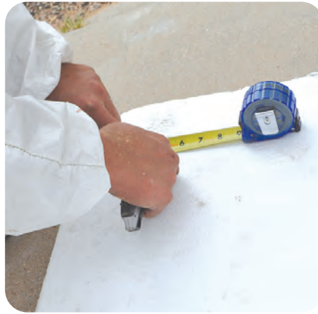
2. Cut blocking material to fit
