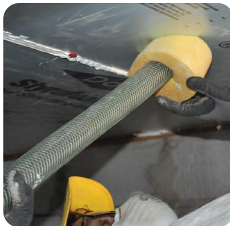
5. Use appropriate fill tube to correspond with work order requirements
