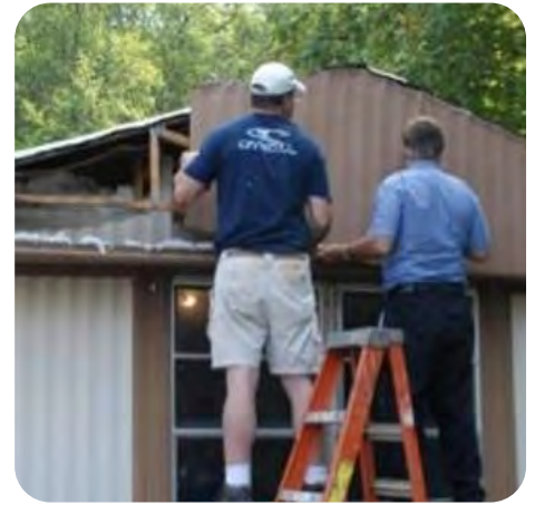
3. Remove or fold up gable end to access attic
