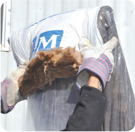
5. Fold batt over end of insulation stuffer
