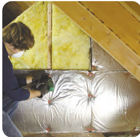
4. Install backing material
