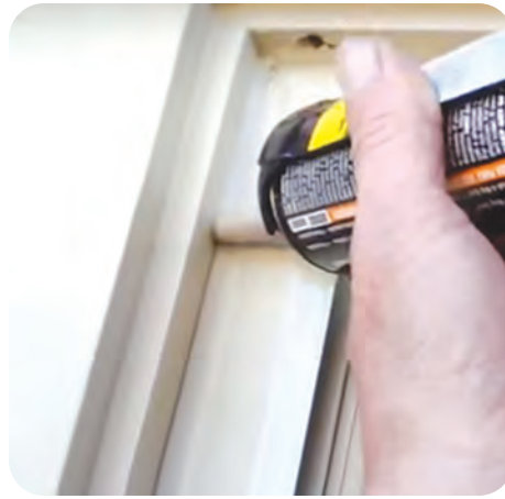
8. Caulk all exterior edges
