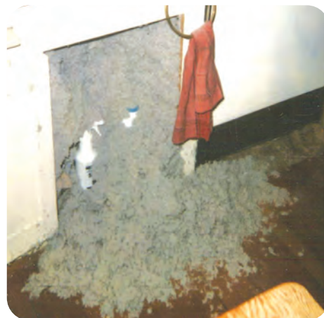
3. Ensure wall integrity is complete (no holes)
