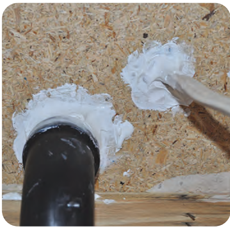
1. Ensure air sealing is complete
