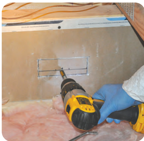
5. Replace access hole plugs in backing material, if possible
