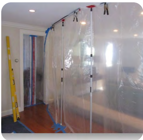
1. Protect work area from debris and dust
