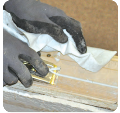
3. Clean up sash or jam and repair any issues
