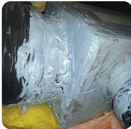
4. Seal new joints
