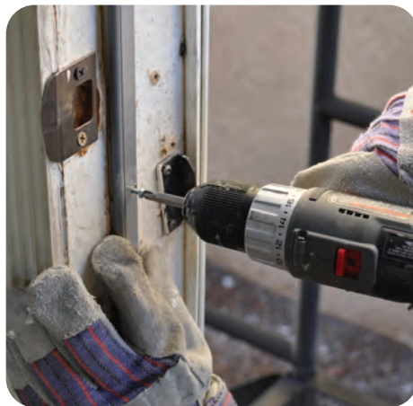
5. Fasten weatherstripping securely when no rabbet exists
