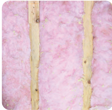
2. Cut batts for exact fit
