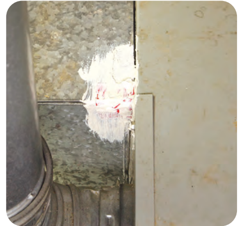
B-3. Apply mastic over the tape
