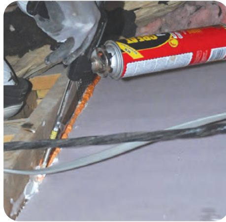
B-2. Seal around infill materials
