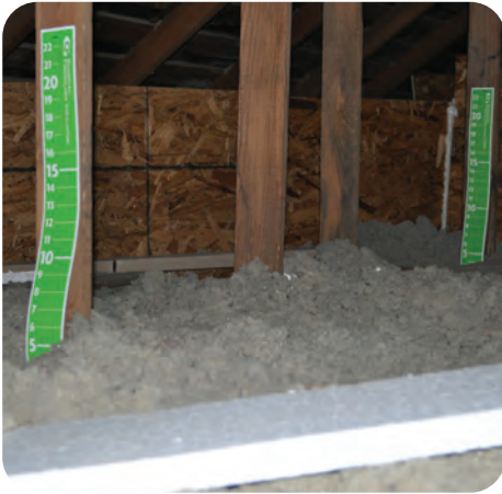
5. Depth rulers installed, 1 per 300 square feet
