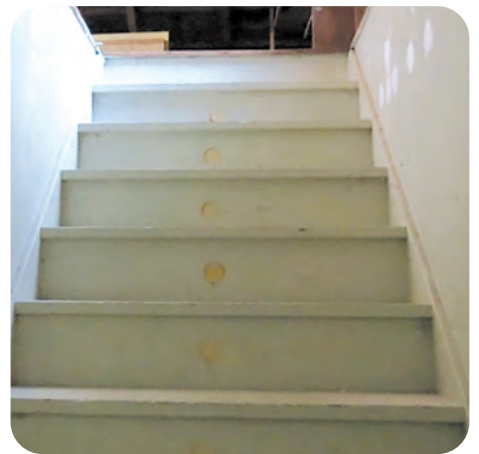
12. Plug access holes from blown insulation
