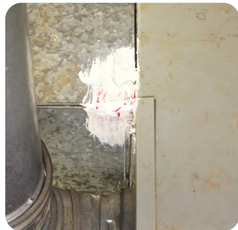
B-3. Apply mastic over the tape
