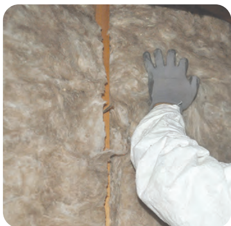
3. Install batts with minimal compression
