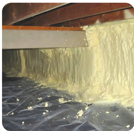
1. Use a fire-rated material
