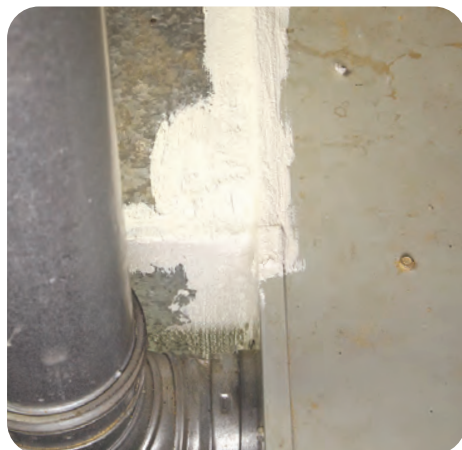
B-5. Apply additional mastic over mesh and tape, extending at least 1 inch past edges of tape in all directions
