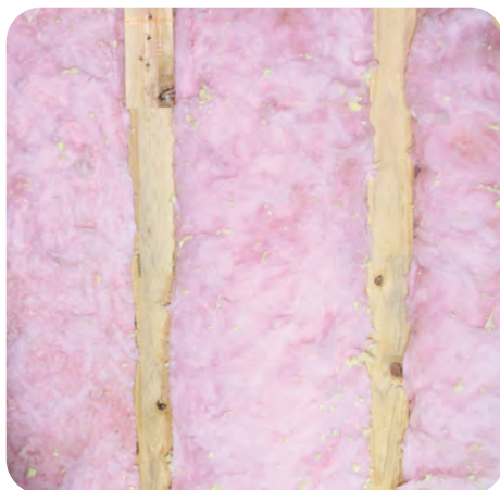
2. Cut batts for exact fit
