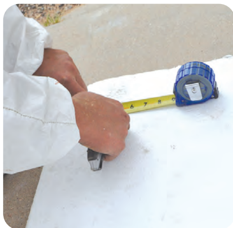
2. Cut blocking material to fit
