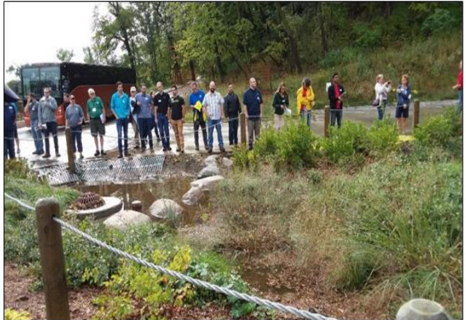
Stormwater infrastructure tour, Omaha
