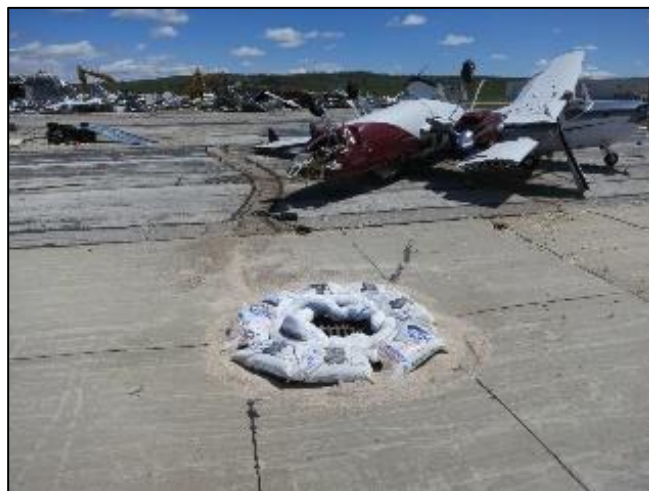
PHOTO 1 – Eppley Airport (April 2024)
