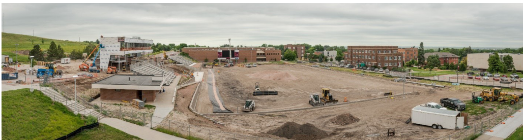
These photos were provided by Chadron State College, which was awarded partial reimbursement of the installation an artificial turf football field. The project was made from 305,000 pounds of recycled tire rubber.
