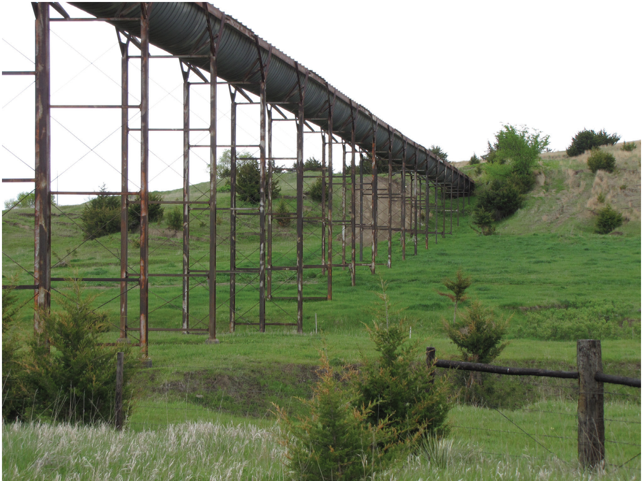
Taylor-Ord canal, property of North Loup Public Power and Irrigation District, located northwest of Elyria, NE.
