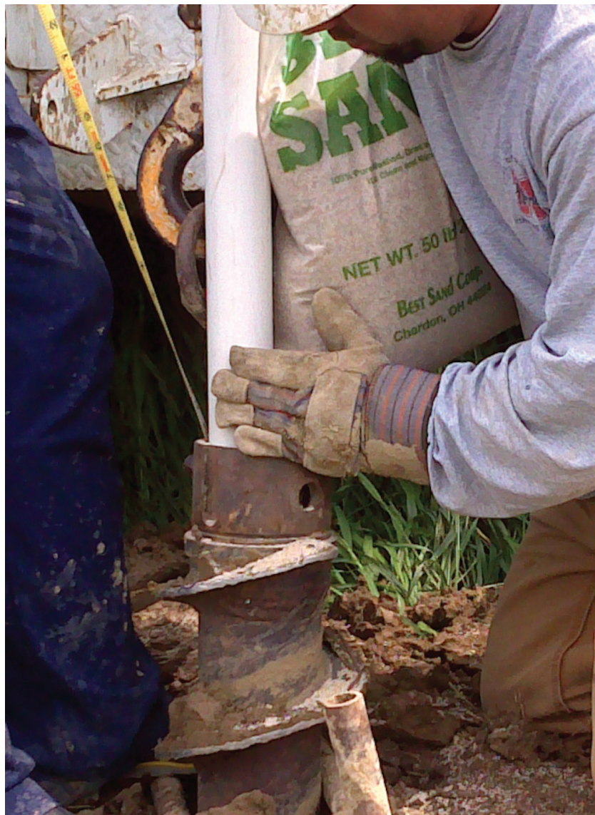
Installing a monitoring well near Clearwater, NE.
