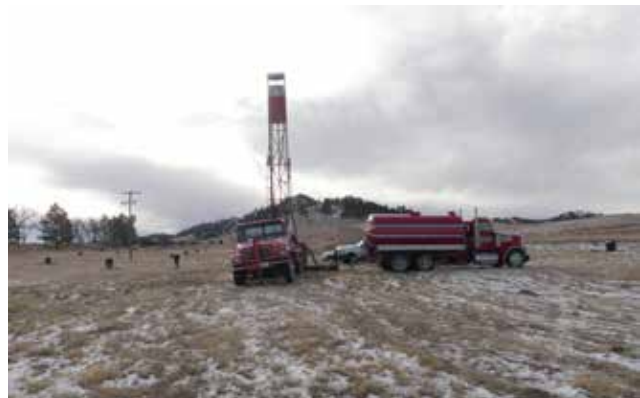
Drilling rig at Crow Butte Resources Inc., Dawes County.
