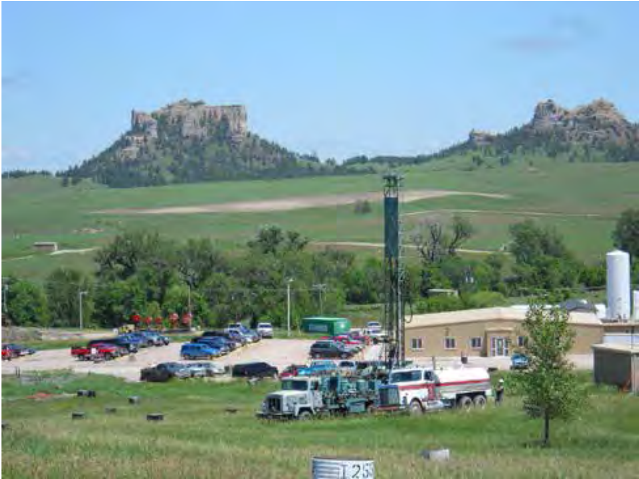
Crow Butte Resources, Inc. in-situ recovery uranium facility. Dawes County.
