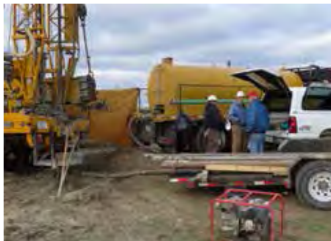
University of Nebraska Conservation and Survey Division (CSD) drilling test holes in the Lower Loup Natural Resources District (NRD) for the design of groundwater monitoring network wells.
