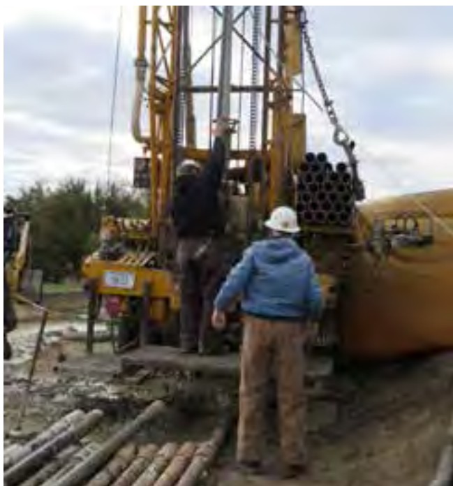
University of Nebraska Conservation and Survey Division (CSD) drilling test holes in the Lower Loup Natural Resources District (NRD) for the design of groundwater monitoring network wells.
