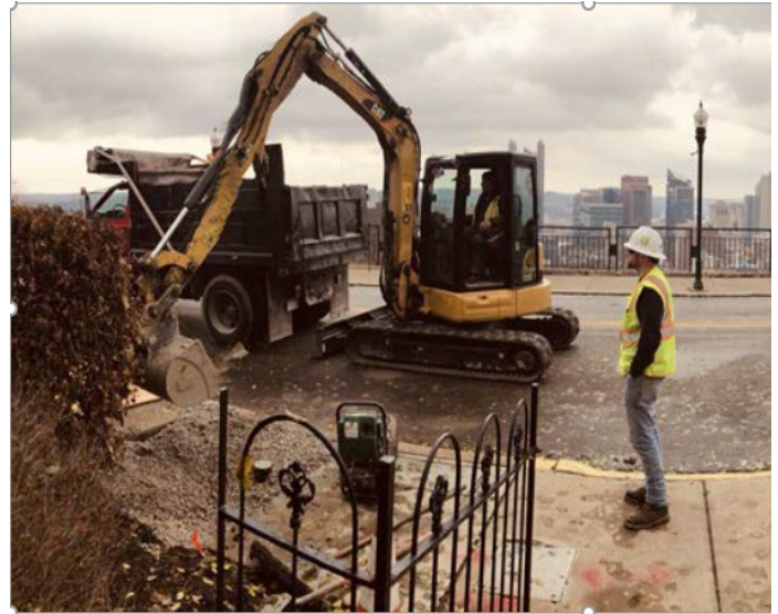
Example of a Mechanical Excavation
