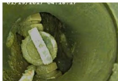
Non-Lead Service Line
