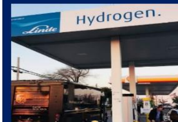
H 2 @Scale H 2 Fueling Station
