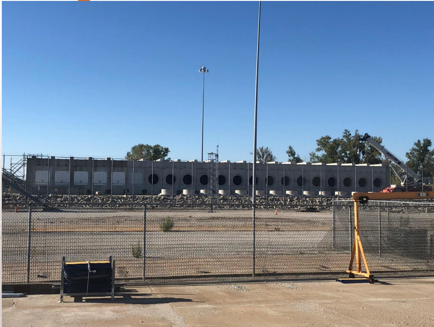
FCS ISFSI – 2018 In Progress
