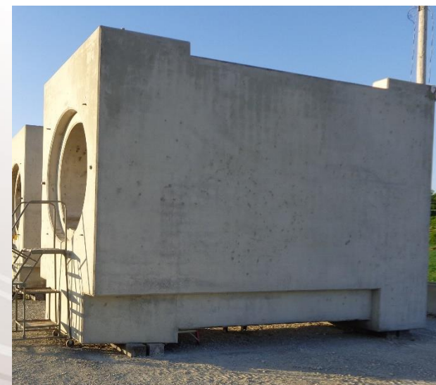
Horizontal Storage Module
