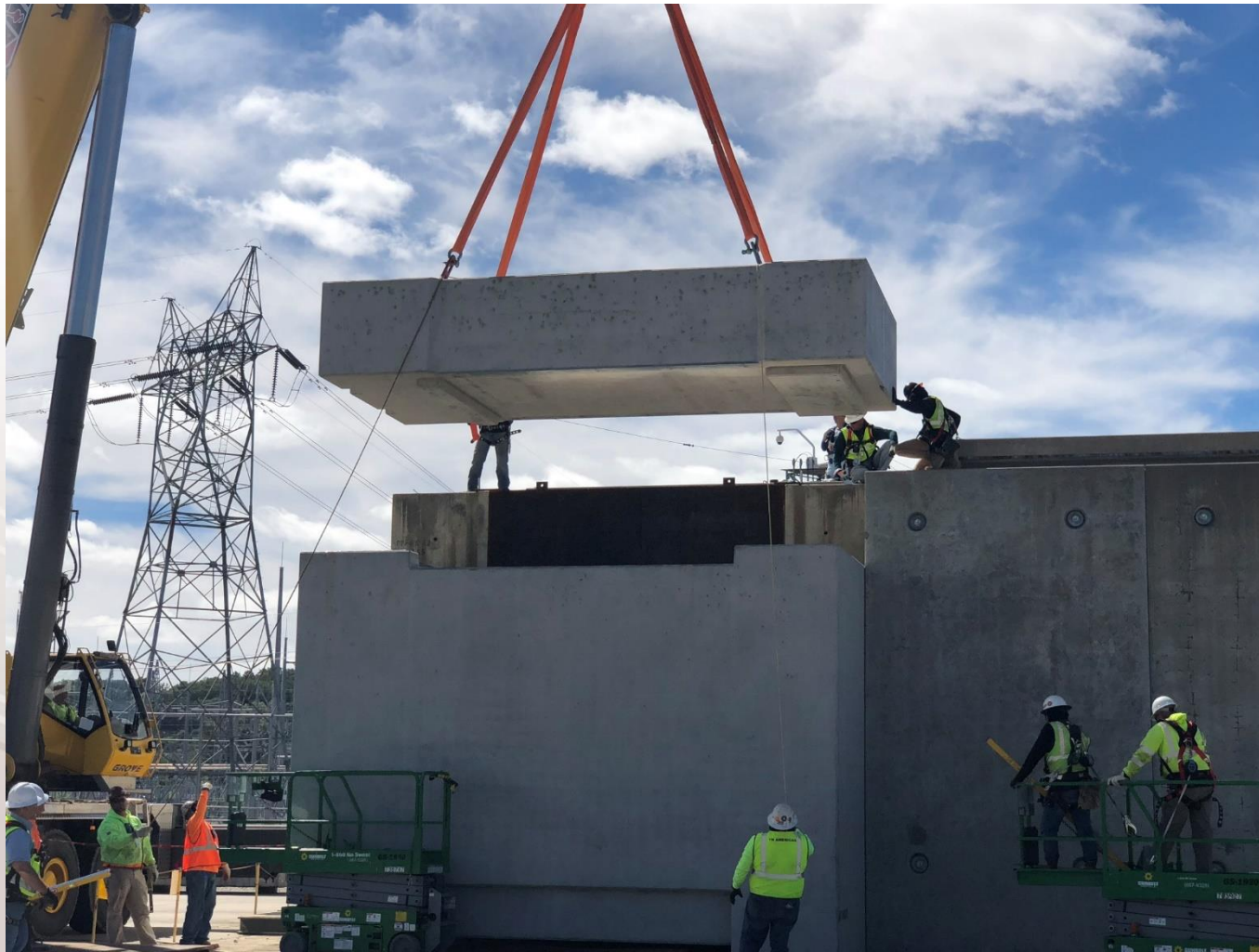
Placing Roof on Horizontal Storage Module
