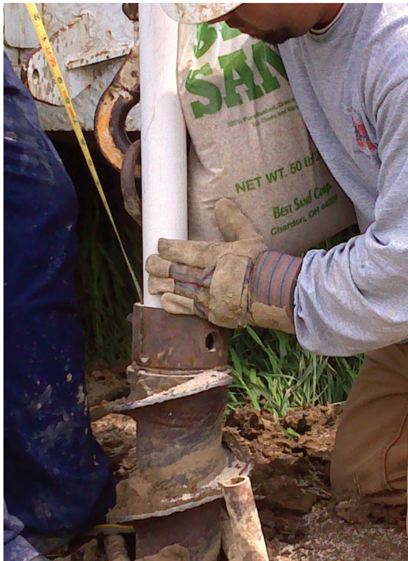
Installing a monitoring well near Clearwater, NE.
