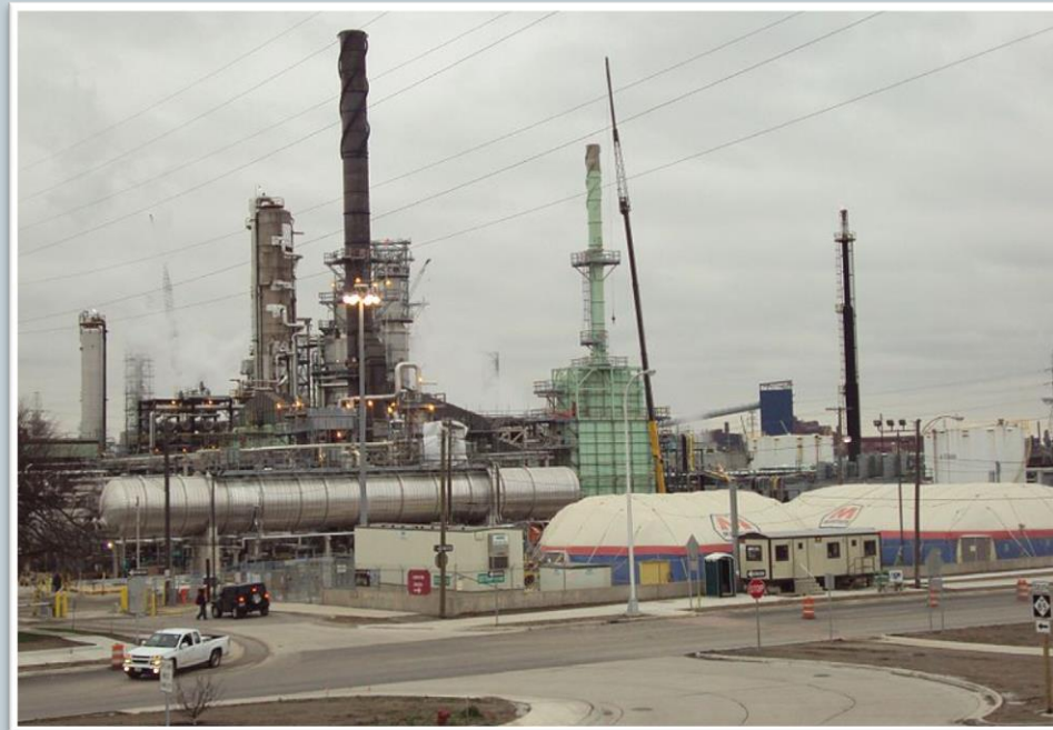
Marathon Petroleum Company (Detroit, Michigan)
