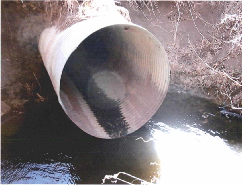
Photo 1. Looking east at culvert on west side of Road 6. Water level is just below the bottom of the culvert pipe. Water is fairly clear, although there may be a darker material along the bottom of the drainage way.
