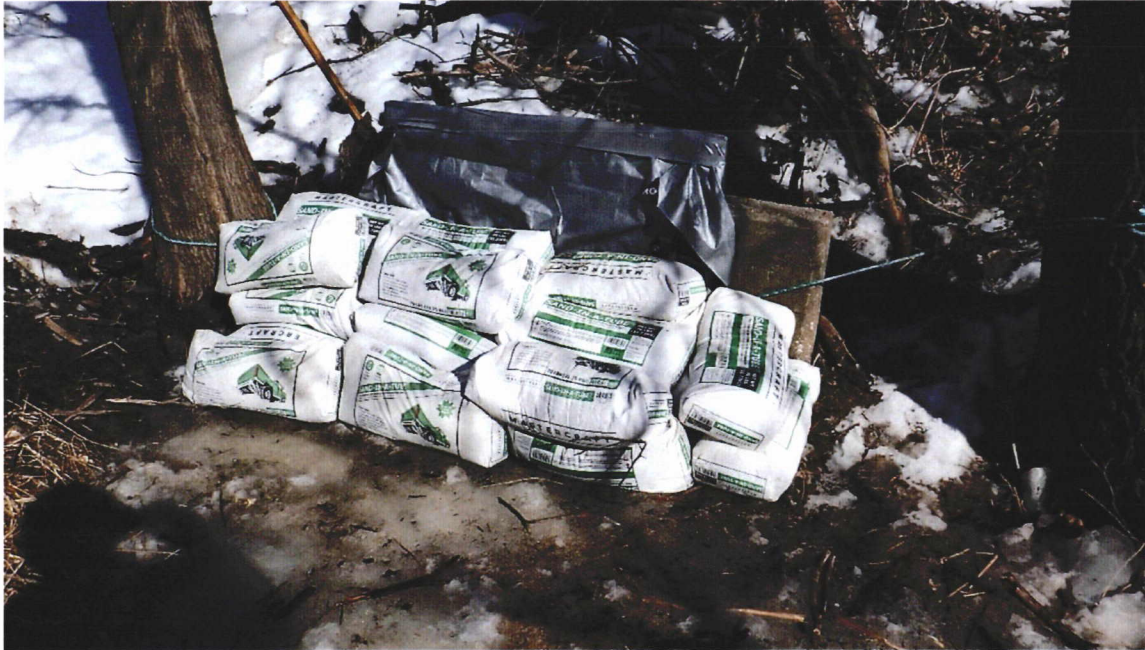
Site 3, west side of Highway 66. Sandbags and tarp-covered plywood blocking the culvert. There is also an inflated packer in the culvert.
