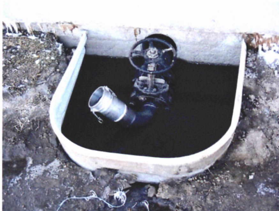
Photo: Digester 1 pipe/valve with standing stillage discharge water.
