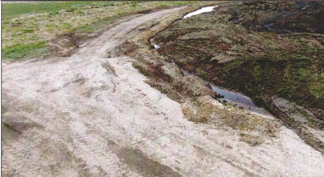
Video: DJI_0878 Date: April 15, 2021 Photographer: D. Pauley Camera: Mavic 2 Zoom Subject: Video of stormwater berm on east and south side of east wet cake piles, looking south
