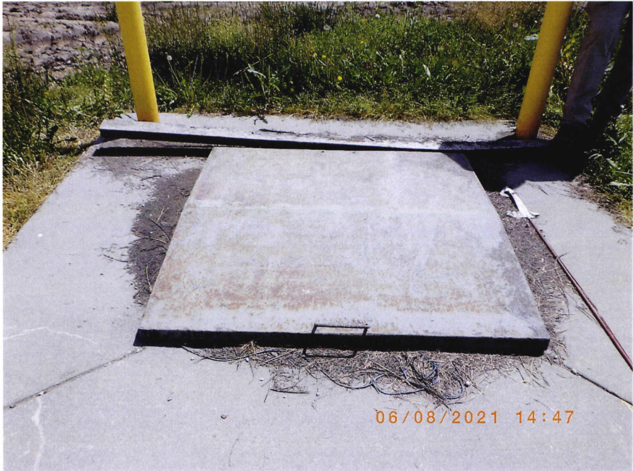
First Tank lid. Lid is secure and undamaged. Mud and plant debris accumulation is consistent with precipitation gathering in the area and is not indicative of/evidence of overflow. Photo taken facing South.
